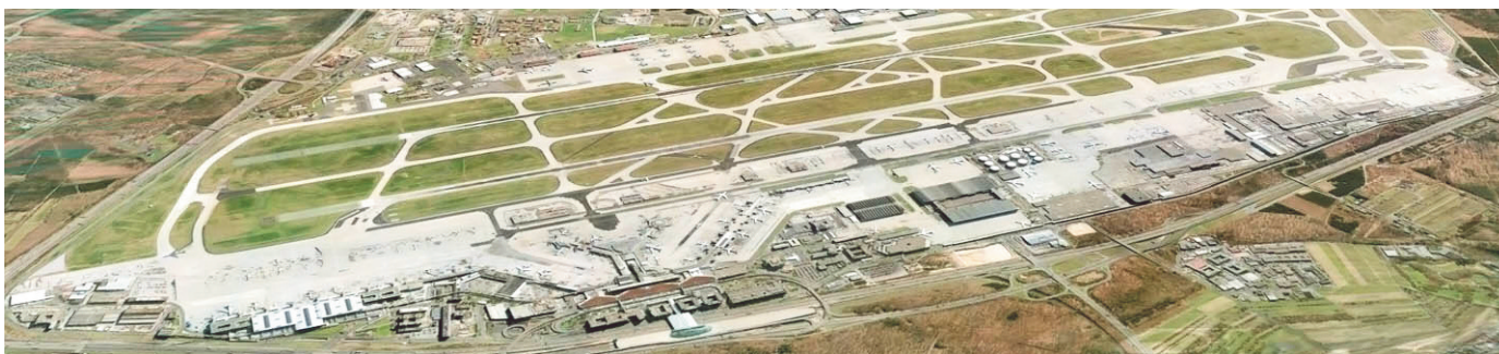
Airport used as a hub
