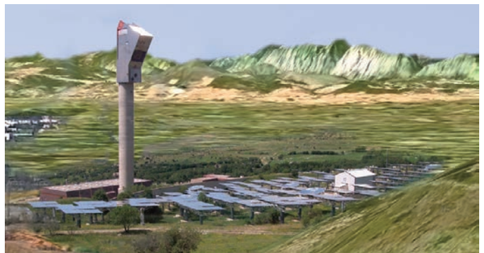
Solar power plant
