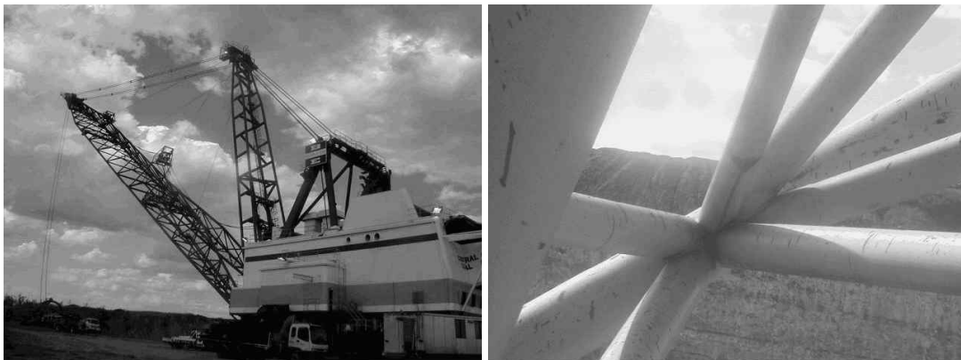
Figure 1: Dragline, and a typical weld cluster
