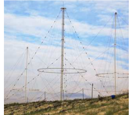
The transmitting antenna array for the surface wave radar, comprising three bi-cone antennas.
